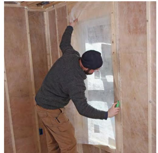
**Trim around doors and windows.** Excess netting is trimmed along the bottom plate and around the perimeter of framed openings where it covers doors and windows. The non-woven material cuts easily with a fresh blade.
