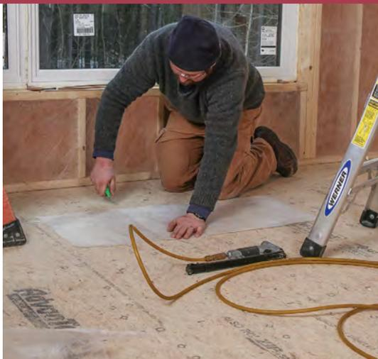
**Cut small pieces on the floor.** Precision isn't critical for the small pieces of netting used to divide cavities, but using a measured piece as a template helps speed the work of cutting a stack of the small rectangles needed to divide the 16-in.-deep rafter cavities.
