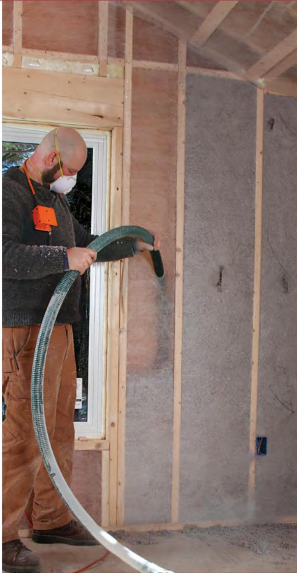
**Fill from the bottom up ...** In an 8-ft. or 9-ft. stud cavity, the whip is inserted near the middle and pushed all the way to the bottom plate. As the cavity fills, the whip is slowly withdrawn. When the cavity is half filled, the whip is removed.
