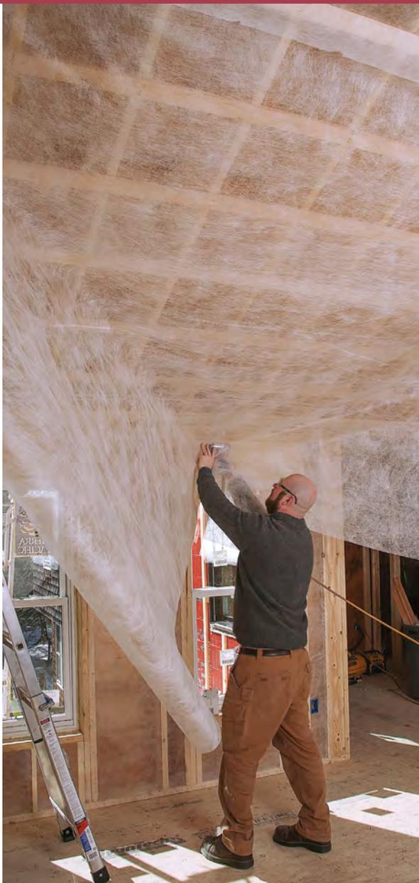
**Drape and pull.** Ceiling cavities are tackled much the same as walls. The netting is fastened to the ridge and allowed to hang down, then pulled tight and fastened along the bottoms of the rafters before lip-stitching.
