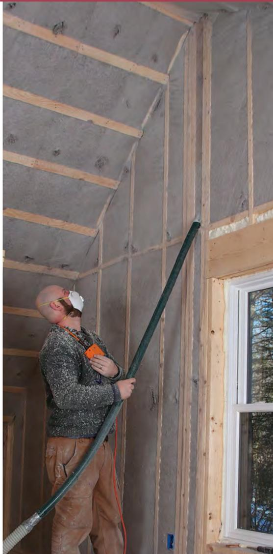
**Beware of blind spots.** Odd-shaped and hidden cavities are marked with a Sharpie during the netting stage so the insulator remembers to fill these spaces. Blind corners created by adjoining walls are best filled through multiple holes spaced a couple of feet apart, with the hose plunged horizontally into the hidden part of the cavity. Cavities smaller than 2 in. are filled with canned spray foam.
