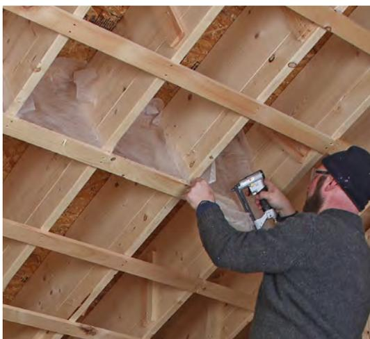
**Divide deep cavities.** Cavities deeper than 12 in. should be divided into cells using small pieces of netting spaced about 6 ft. o.c. The smaller space makes it easier to reach all corners, ensuring the cellulose is installed at the correct 3½-lb.- to 4-lb.-per-cu.-ft. density.
